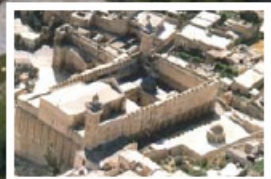
From the north-east
